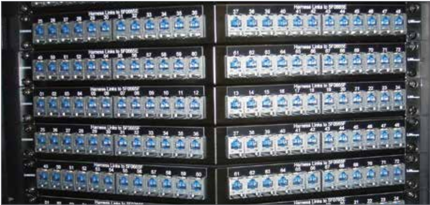
19-in 1U HD Copper Panel with 48 Ports
